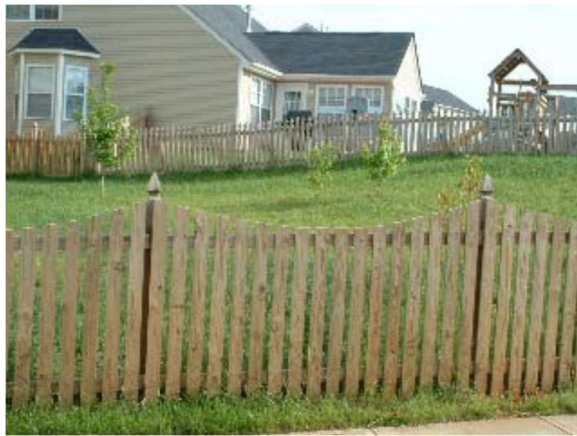
Crescent top fence
