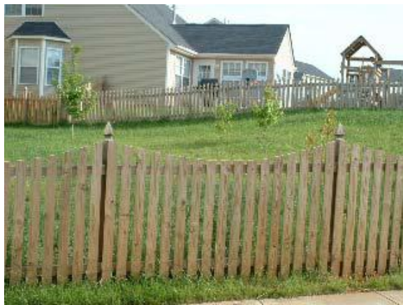
Crescent top fence
